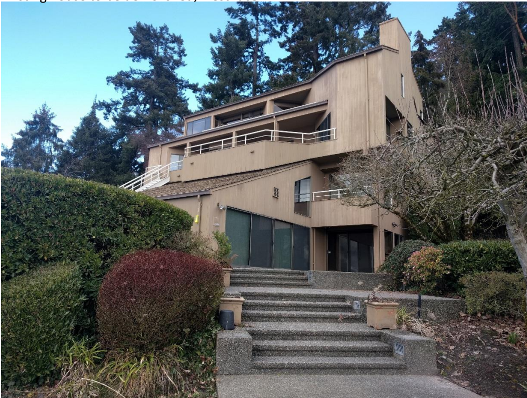
Existing house to be demolished, south face
