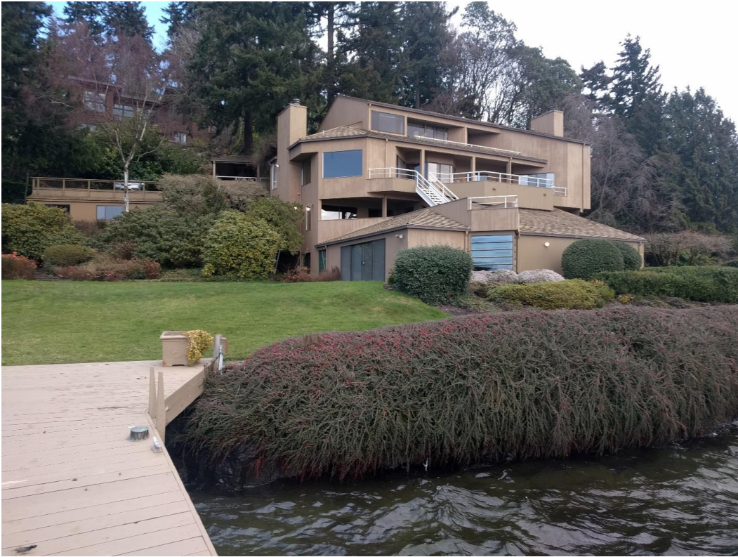
Existing house to be demolished, west face
